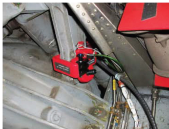
Aft bridge removal
